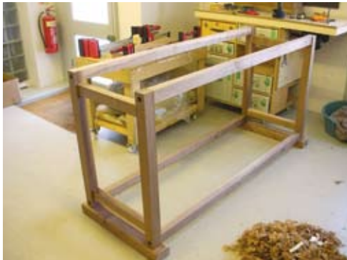
1 The main frame lacks cross bracing as this will come from the cupboards that fit below the worktop
