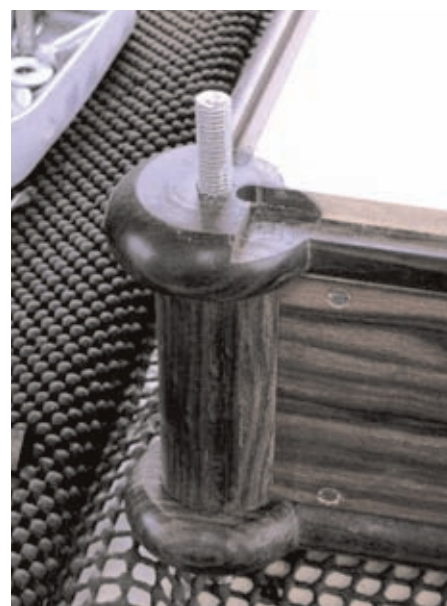
2.2 The corner joint: the channel for the glass is a 4mm continuation recess below the rebate, see drawing
